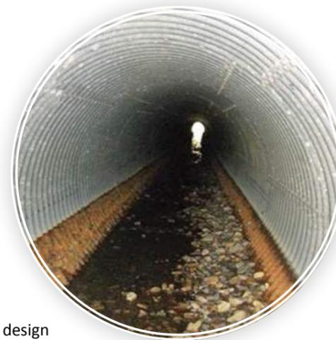
The project involved the rehabilitation of a 100m long 2300mm corrugated steel plate culvert under the Hume Highway at Broadford in Victoria.
